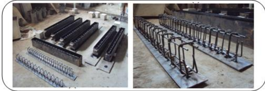
Plate 2: beams fabrication
