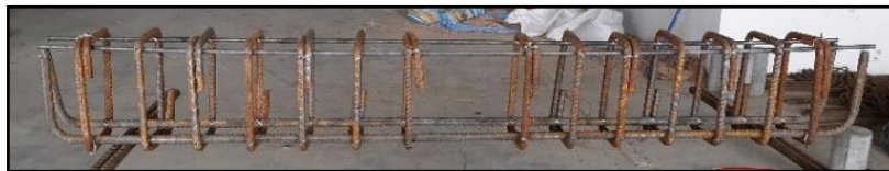
d) Steel reinforcement
