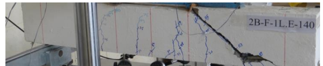
Figure 17 Cracks pattern of beam 2B-F-1L.E-140
