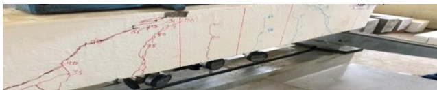
Figure 12 Cracks patterns of beam 3B-S-140
