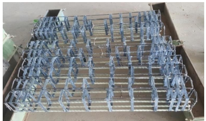
Figure 5 Beams reinforced with CFRP sheets immersed by sikadur330
