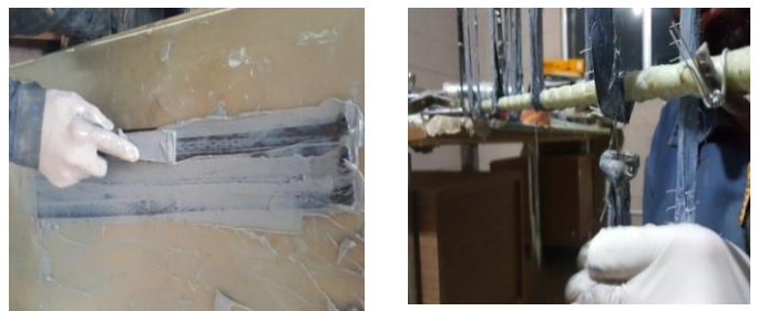
Figure 4 The steps of preparing stirrups with CFRP sheets
