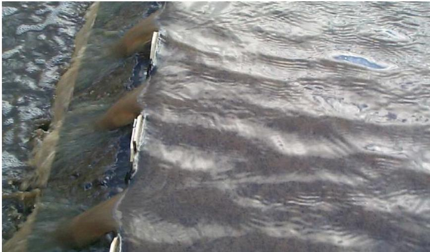
**Plate 3. Overloaded clarifier operations.**
