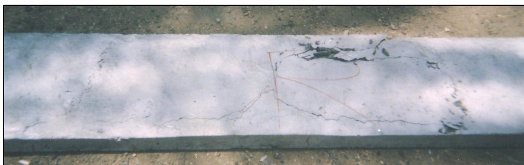
Figure (5) Crack Patterns for tested specimens (bottom face)
