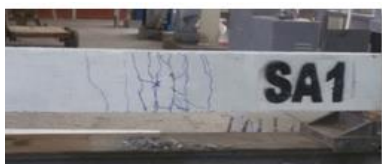
Figure 8.1: Cracks Pattern of Specimen SA1
