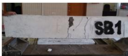
Figure 8.2: Cracks Pattern of Specimen SB1
