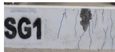
Figure 8.3: Cracks Pattern of Specimen SG1
