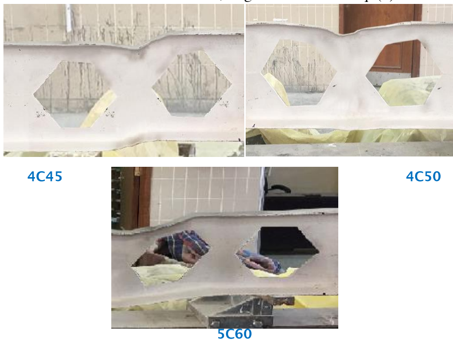
Figure (8) Castellated specimens failing Vierendeel mechanism
